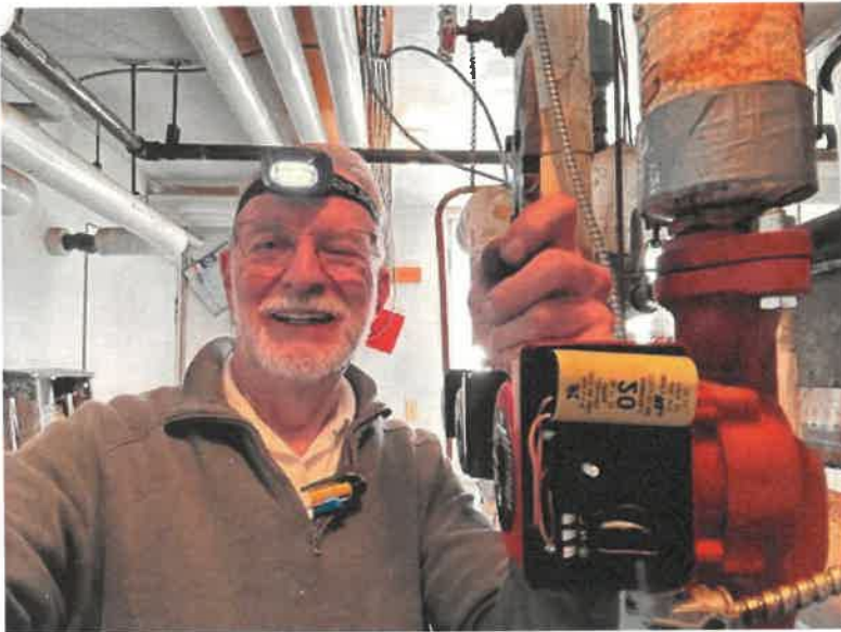
Andrew MacAdam services the pumps in the boiler room.
